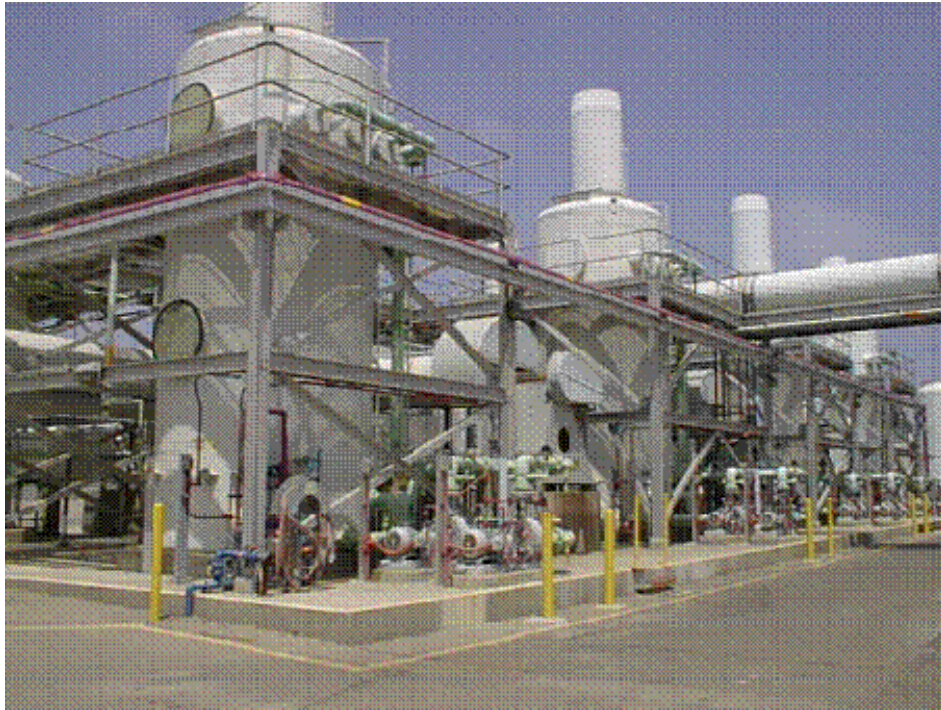
Figure 1. Photo of a bank of eight wet scrubbers at Plant 2 of OCSD. The second from the left has been converted to biotrickling filter Q.
