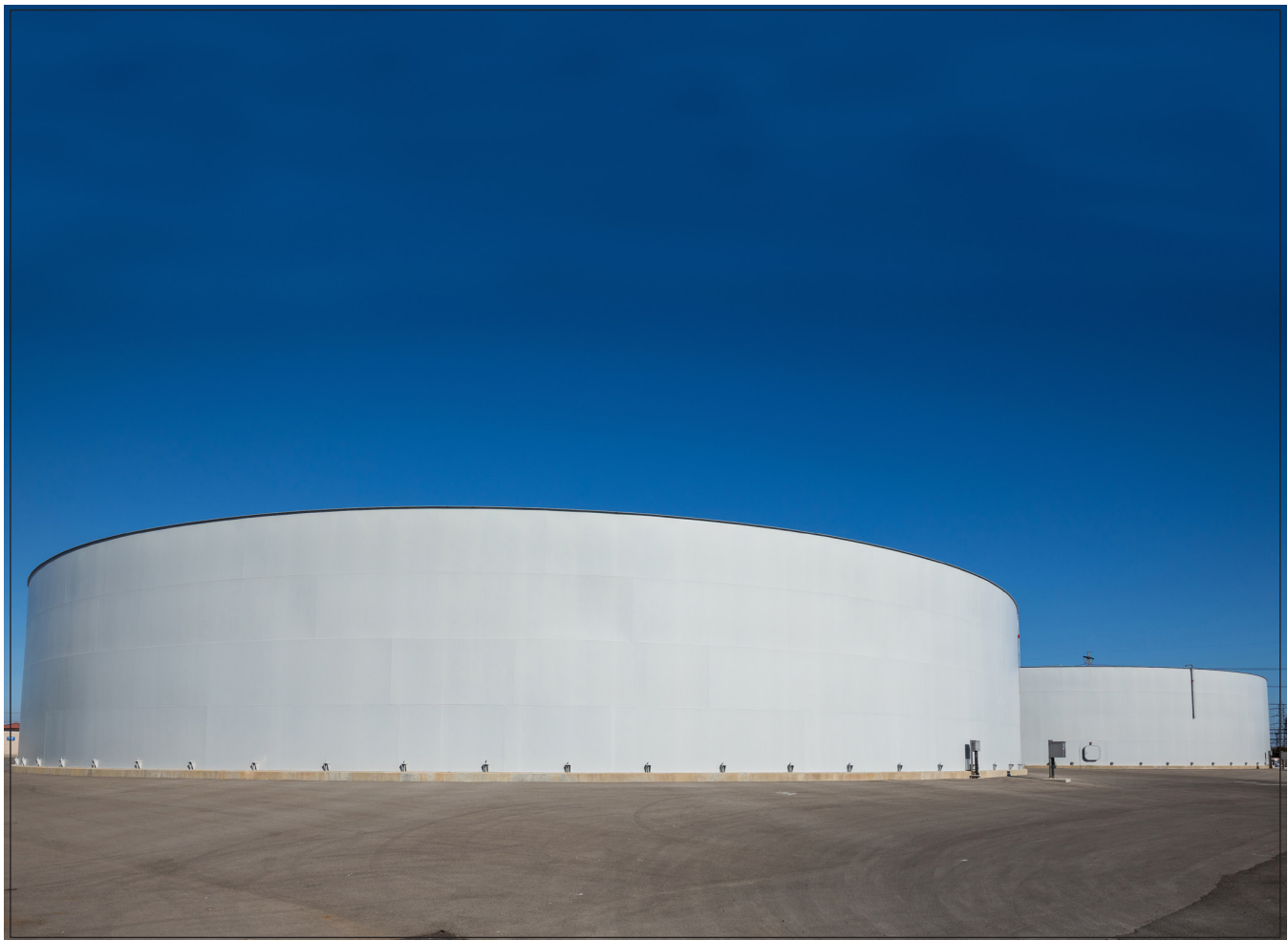
GWRS water tanks at Reclamation Plant No. 1 in Fountain Valley.
