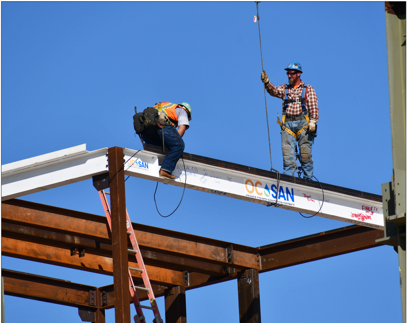
Final steel beam installation at Headquarter Complex.
