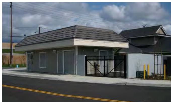
The completed College Pump Station fits in with residences in the neighborhood.
