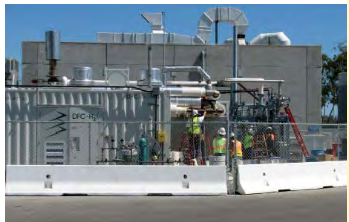
Fuel cell pilot study installation – this technology could potentially replace the central power generation system engines, thus reducing air emissions while producing power, heat, and hydrogen fuel.
