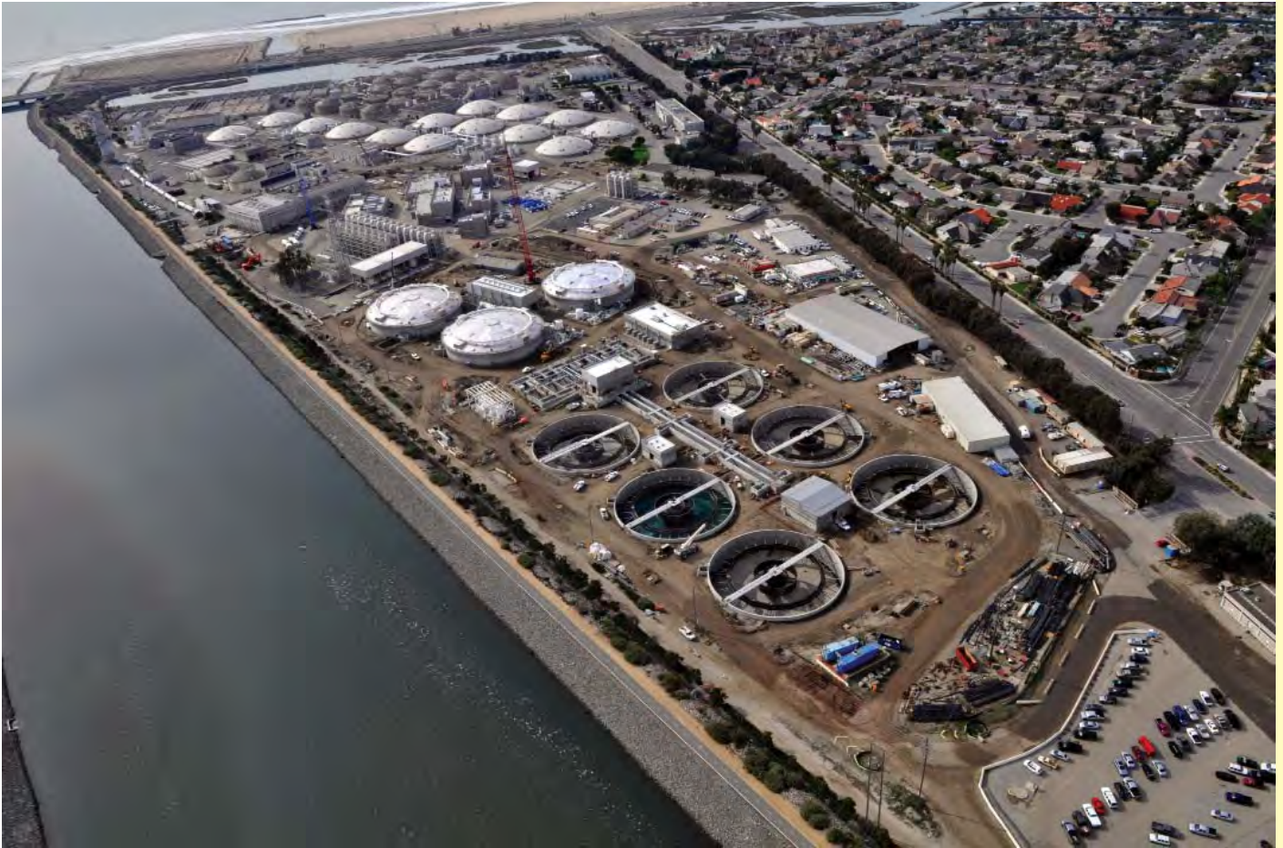
OCSD's Treatment Plant No. 2 spans 200 acres and borders Brookhurst Street, the Santa Ana River, and Pacific Coast Highway in Huntington Beach, CA.
