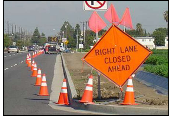
Figure 1: Traffic Control, Lane Closure (typical)
