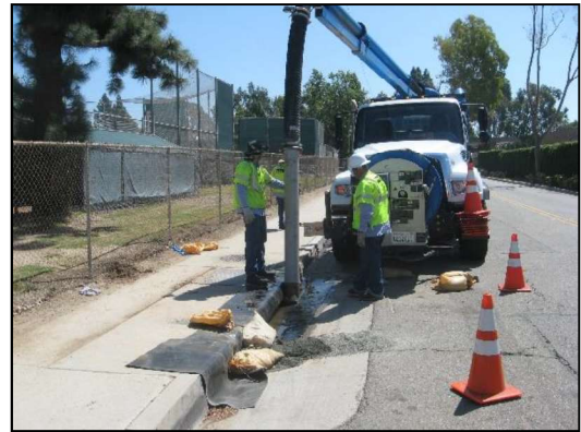
Figure 4: Overflow Clean Up Using Industrial Combination Sewer Cleaning Vehicle (typical)
