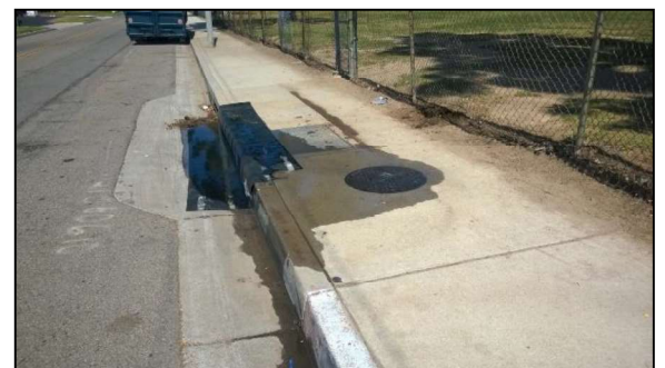
Figure 3: Spill Containment Set-Up (example)
