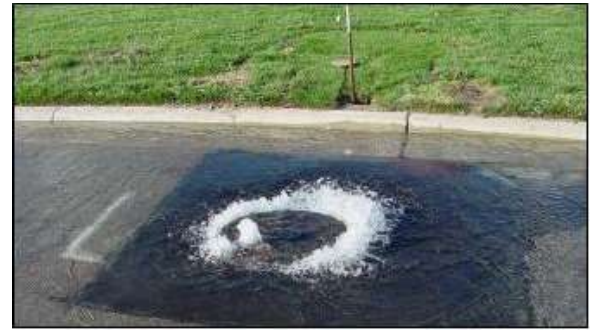
Figure 2: Overflowing Manhole (example)
