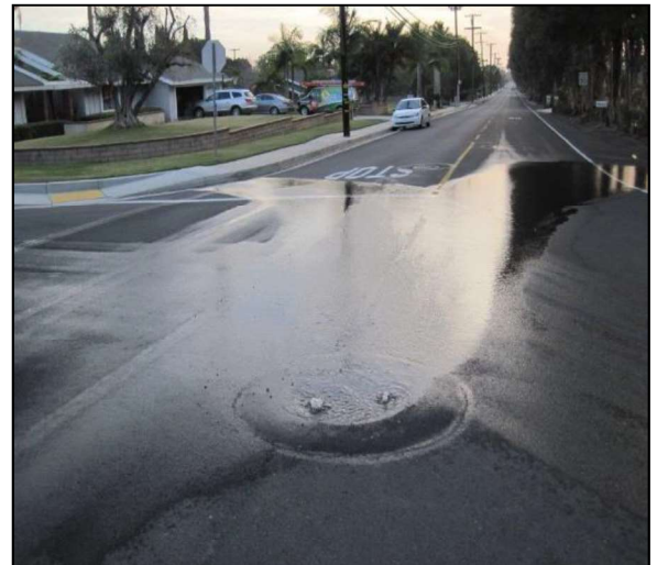
Figure 6: Spill Area Documentation Photo (typical)
