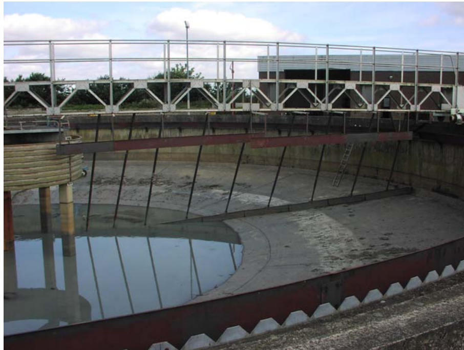
Figure 3.2 Primary Basin prior to ABR retrofit
