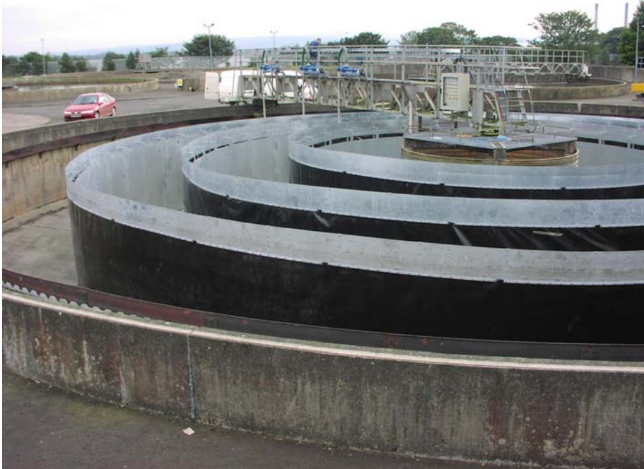
Figure 3.3 Primary basin following ABR retrofit - note the three sets of baffles
