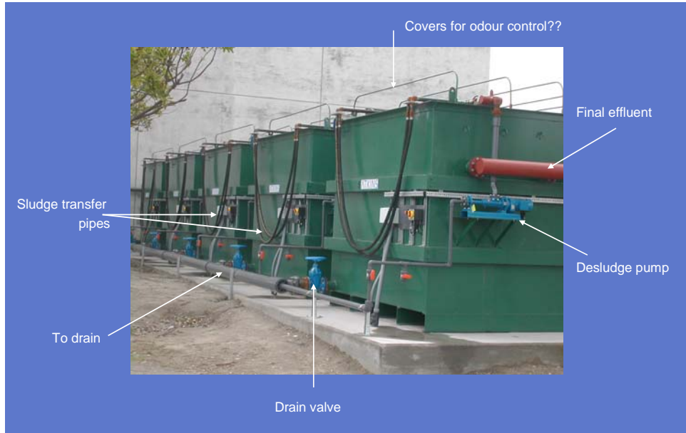
Figure 4.1 Tank overview; 5 compartments
